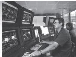
Intelligent Building Management
